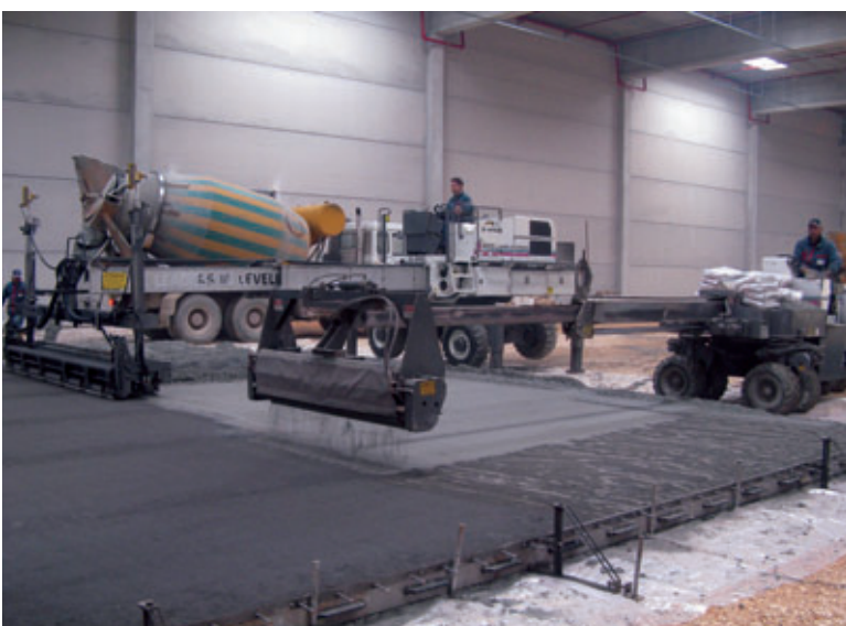
Owens Corning Alkali Resistant glass fibers deliver superior performance reinforcement for concrete industrial flooring.
