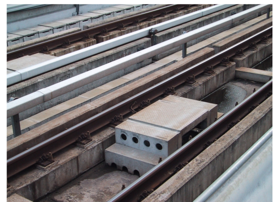
GRC Evacuation Bridge
