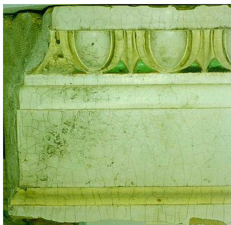
Structural and surface deterioration of the original terracotta
