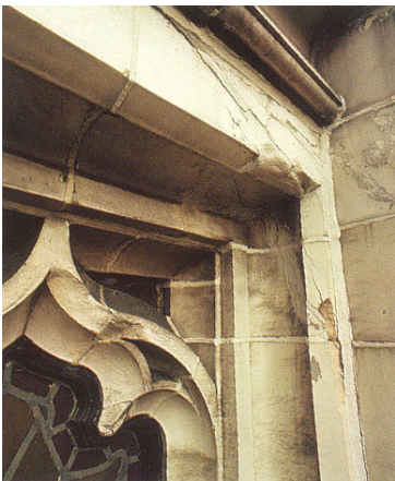
Structural and surface deterioration of the original terracotta
