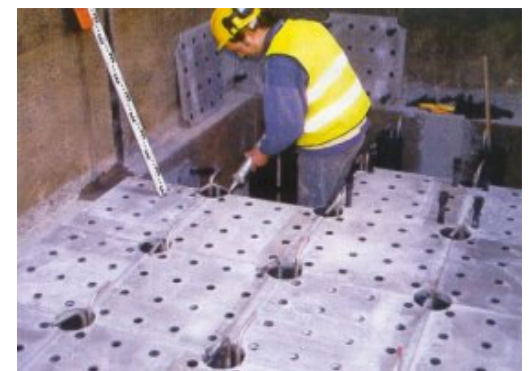
Joints sealed with mastic
