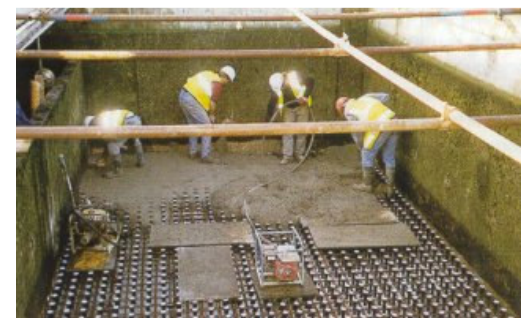
Pouring and levelling of concrete
