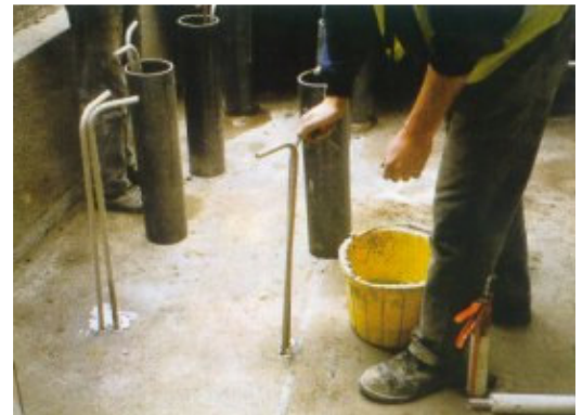
Anchor bars fixed with epoxy
