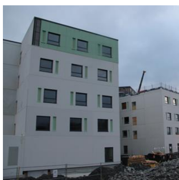
Precast insulated façade panels in place
