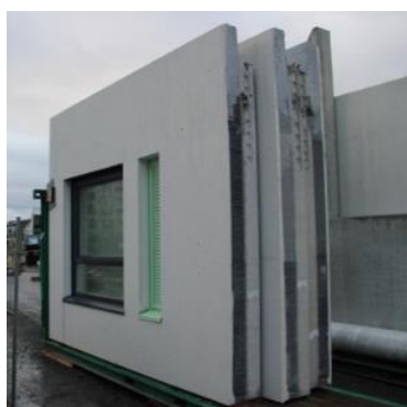
Precast insulated wall panels delivered to site with integrated windows and blinds
