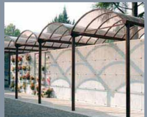
Bosisio Ltd. (Italy) created a modular system with fiberglass panels that can assemble 100 crypts in a few days.
